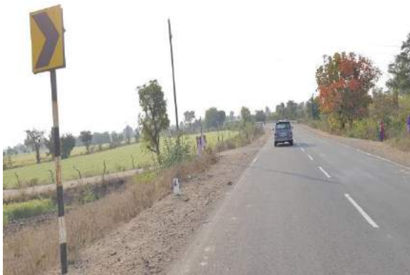
Km. 30+100 – Road Marking
